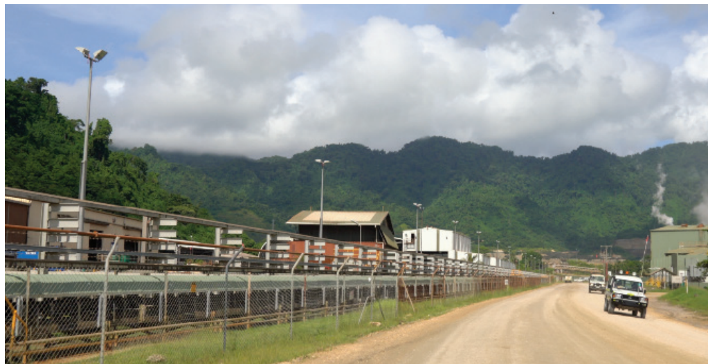
Lihir gold mine conveyor, Lihir Island. Source: Tim Grice
